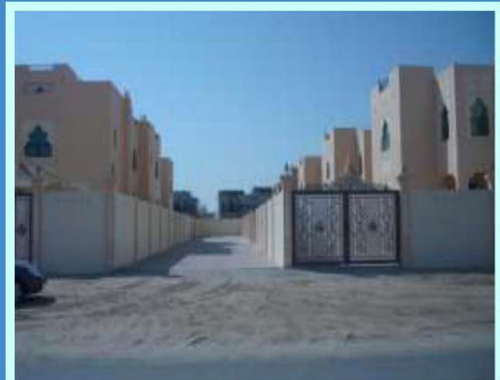
SECTOR : 12 VILLA COMPOUND MBZ CITY SCOPE : SUPPLY & INSTALLATION OF GLASS WINDOWS & DOORS, HANDRAILING
