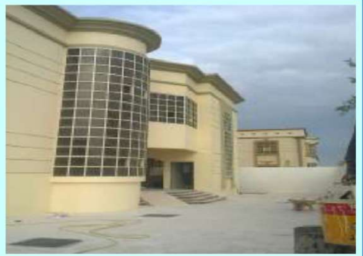
SECTOR : Z15, PLOT : 40 MBZ CITY SCOPE : SUPPLY & INSTALLATION OF GLASS DOORS , WINDOWS
