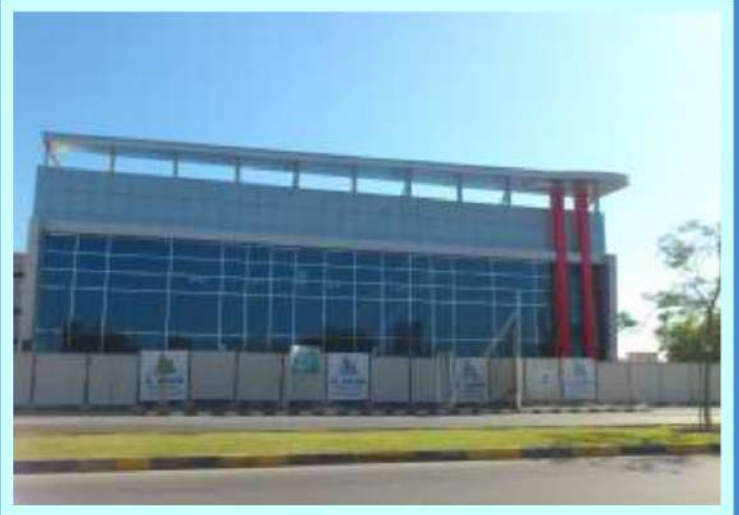
SECTOR : SHOWROOM MUSAFFAH, SCOPE : SUPPLY & INSTALLATION OF GLASS CURTAIN WALL & WINDOWS
