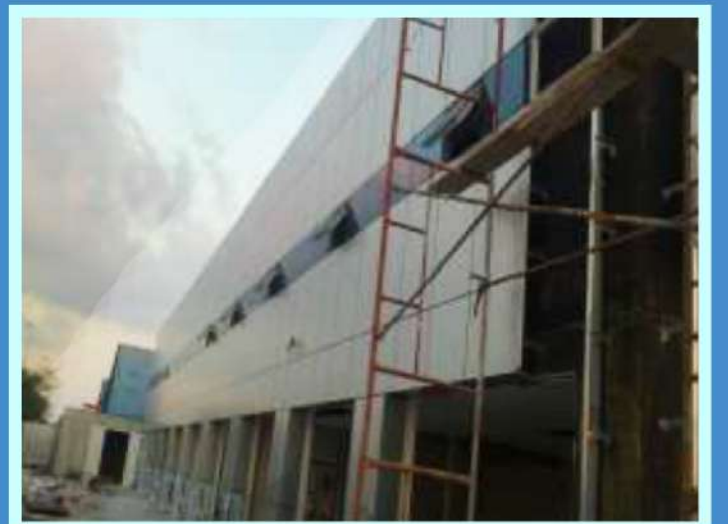
SECTOR : M14 MUSAFFAH COM BUILDING SCOPE : SUPPLY & INSTALLATION OF EXTERNAL ACP CLADING & WINDOWS
