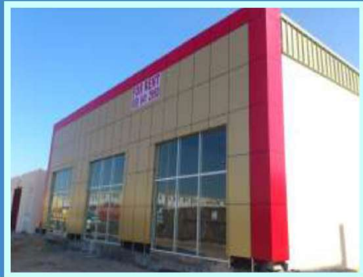
SECTOR : M40 MUSAFFAH COM BUILDING SCOPE : SUPPLY & INSTALLATION OF EXTERNAL ACP CLADING & WINDOWS
