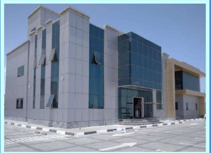
SECTOR : M38 MUSAFFAH COM BUILDING SCOPE : SUPPLY & INSTALLATION OF EXTERNAL ACP CLADING & GLASS CURTAIN WALL
