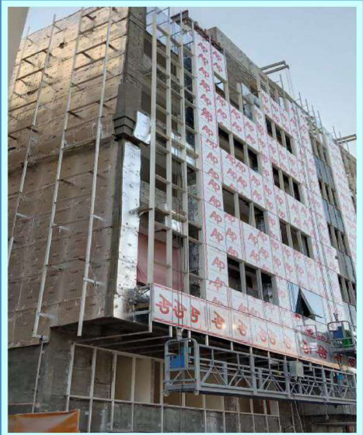
SECTOR : MORROR , ABU DHABI SCOPE : SUPPLY & INSTALLATION OF GLASS CURTAIN WALL AND ACP PANEL,
