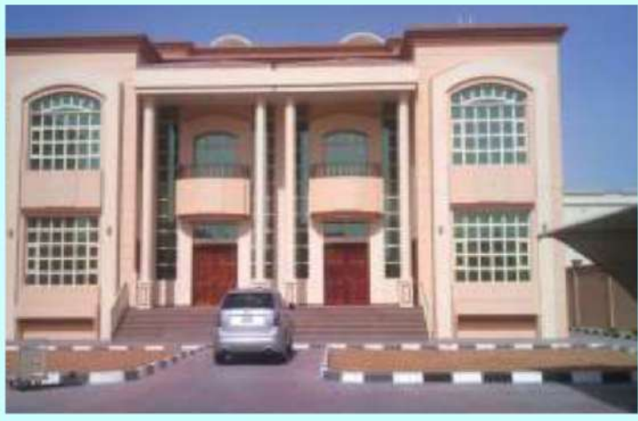
SECTOR : Z29, PLOT : 21 MBZ , CITY SCOPE : SUPPLY & INSTALLATION OF GLASS DOORS , WINDOWS & HAND RAILING
