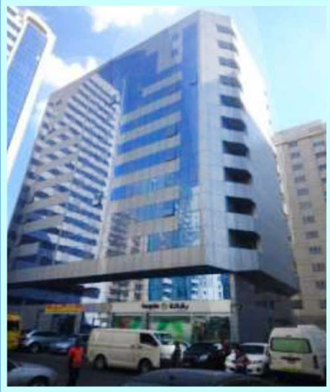
SECTOR : E13 , BUILDING : 18, TCA SCOPE : SUPPLY & INSTALLATION OF EXTRANAL GLASS CURTAIN WALL AND ALUMINIUM ACP PANEL CLADDING
