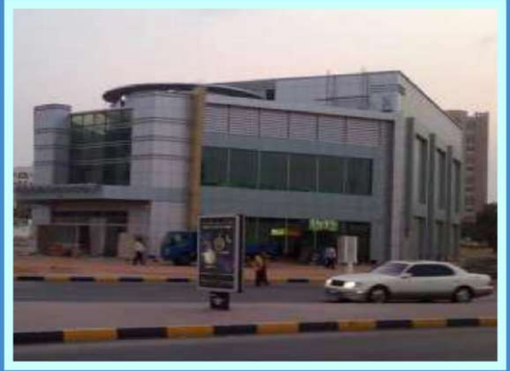
SECTOR : NATIONAL HYPERMARKET, FUJAIRAH SCOPE : SUPPLY & INSTALLATION OF GLASS CURTAIN WALL & WINDOWS
