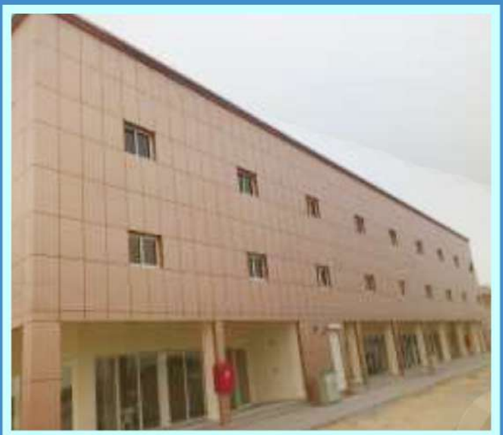
SECTOR : MUSAFFHA M40 PLOT : 17 SCOPE : SUPPLY & INSTALLATION OF DOORS WINDOWS AND EXTRANAL ALUMINIUM ACP PANEL CLADDING
